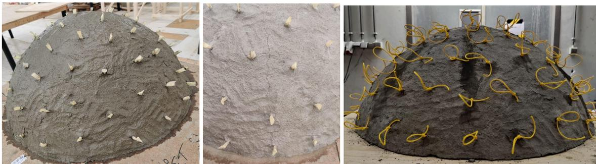
Figure 2.3.4: a) Dome covered in wet concrete. b) Crack in dried concrete. c) Patched up cracks
