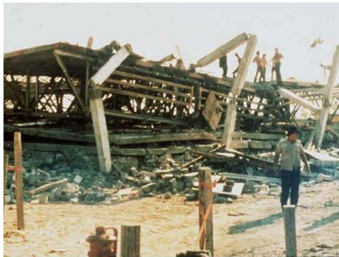
Figuur 4: Harbour Clay Condominium ingestort 3
