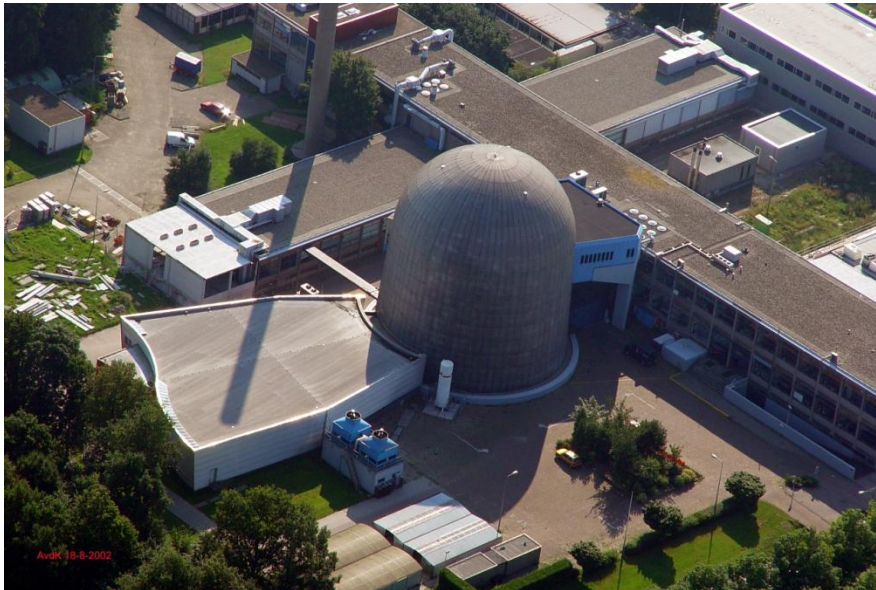
Figure 6: Reactor Institute Delft
