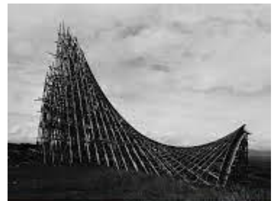
Figure 6 Falsework of the shell of the Chapel Lomas de Cuernavaca, Mexico, 1959, by Félix Candela et al. From "Design process for prototype concrete shells using a hybrid cable-net and fabric formwork" (Veenendaal & Block, 2014)
