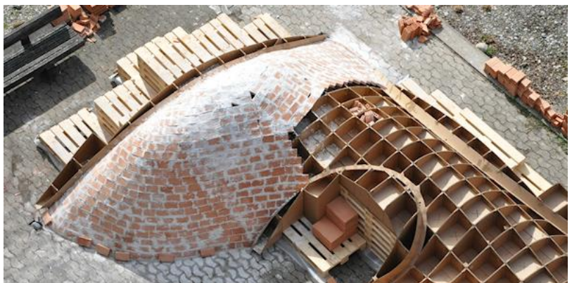
Figure 9 Timbrel Vaulting Using Cardboard Formwork by M. Rippman et al. From "No Tech magazine" (De Decker, 2011)
