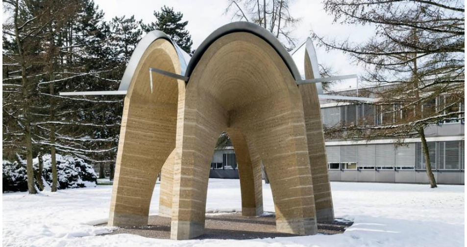
Figure 21 Prefab rammed earth vault, Zürich, Switzerland. From “Block Research group” by Gian Salis, 2014 ( https://block.arch.ethz.ch/brg/teaching/rammed-earth-vault )
