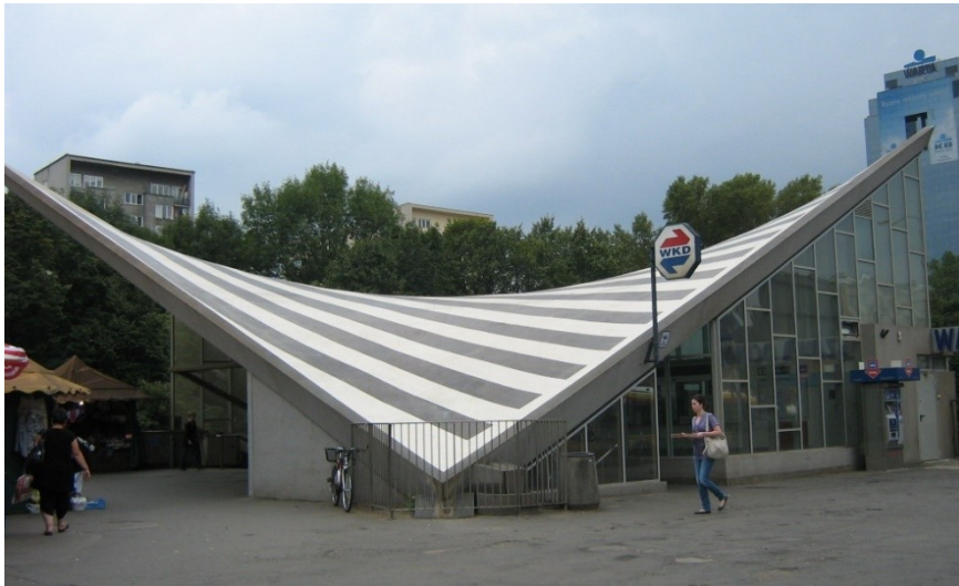
Figuur 1.1: Hypar Dak, Station in Polen, Warszawa Ochota (Bron: Wikipedia pagina: 'Saddle Roof')
