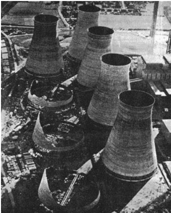
Figuur 1: Three collapsed cooling towers at Ferrybridge, UK [ http://homepage.tudelft.nl/p3r3s/CT4143_handout_15.pdf ]
