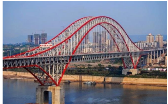
Figuur 5. Chaotianmen bridge, China. (Prandi, n.d.)
