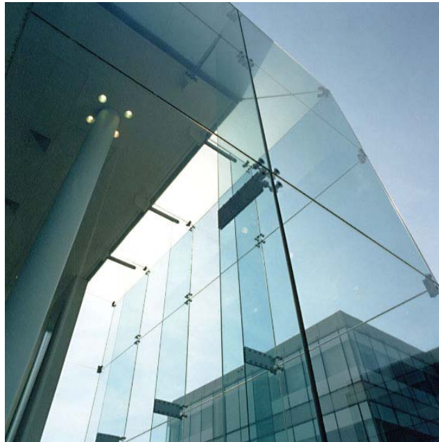
Structural glazing in the Heinz Building Stockley Park, West London, Architect T.P. Bennett
