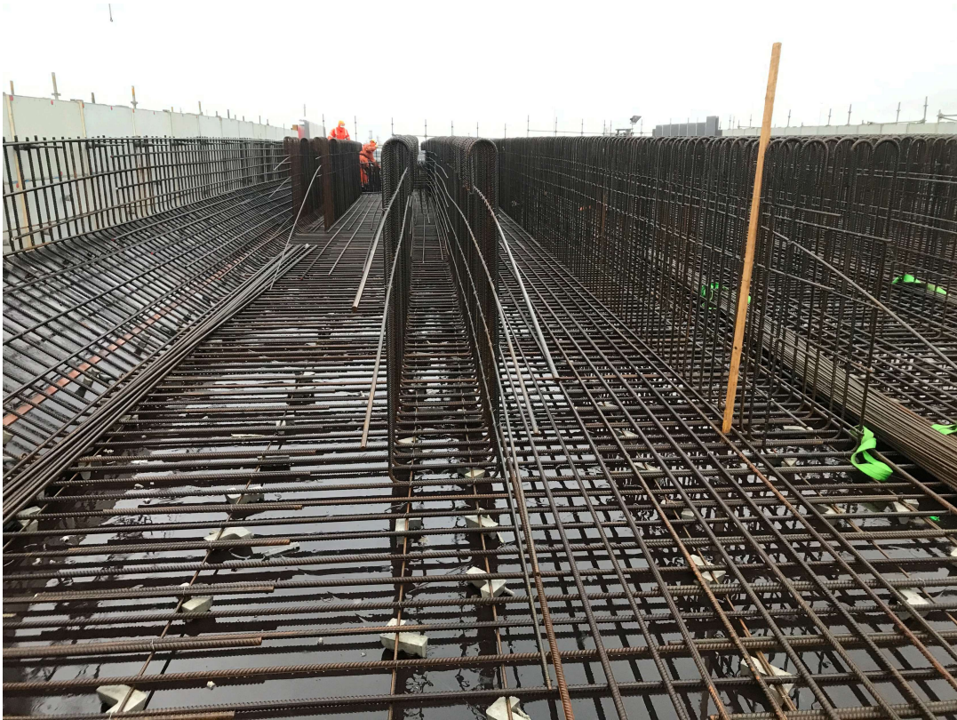
Figure 2.5: Transverse, longitudinal and shear reinforcement
