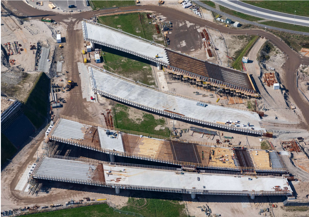
Figure 1.3: Top view bridge decks under construction (March 2021)
