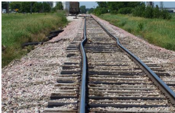
Figure 1.1: Deformed rail, (Globe Gazette, n.d.)
