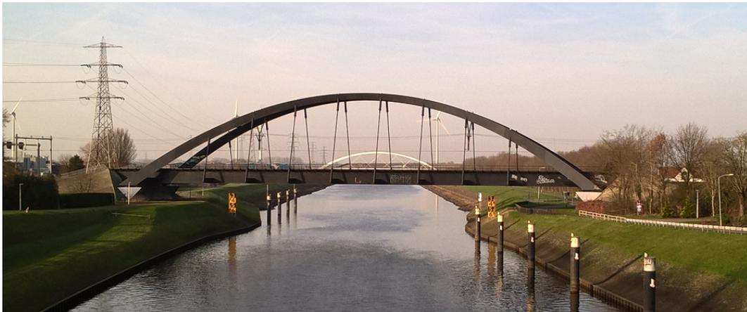
**Figure 4.1:** Spoorbrug Twentekanaal with hanger inclination clearly visible.
