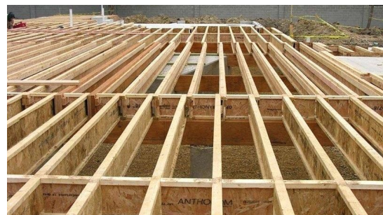
(b) I-joists as beams for flooring [33]
