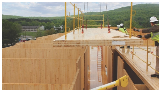
(a) CLT floor panel hoisted on top of CLT walls [25]
