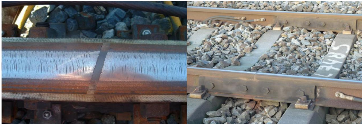
Figure 1.1: (left) IRJ in Australia at 15 degrees (Mandal, 2010); (right) square cut IRJ in the Netherlands (ProRail, 2019)
