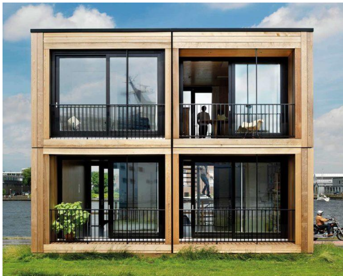
Figure 46 - Finch Buildings modular timber unit [51].
