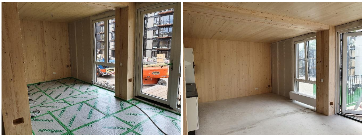
Figure 93 - Units before and after the cement screed is placed, left to right respectively.
