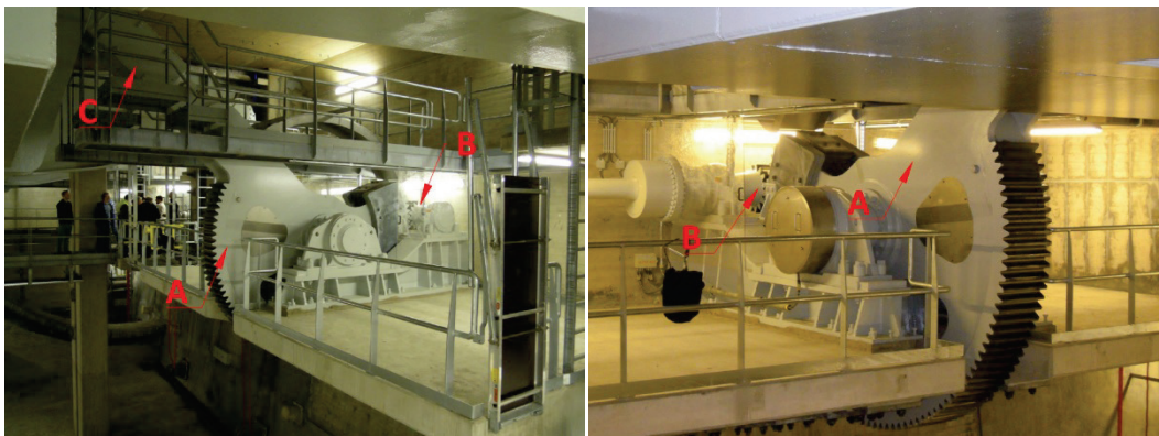
Figure 2.5 - Operating mechanism in Ketelbrug, The Netherlands A: panamawheel, B: pinion, C: push-pull rod
