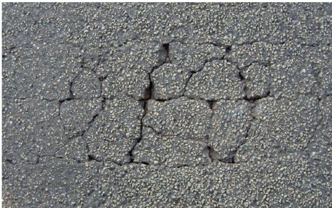
Figure 1.4 Cracks in the asphalt layer, possible indicating deck plate cracks
