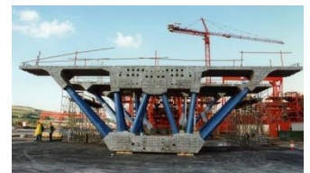
FIGURE 8-3 SECTION OF ECHINGHEN VIADUCT [36]
