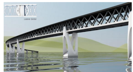
FIGURE 9-4 LATTICE BRIDGE GIRDERS
