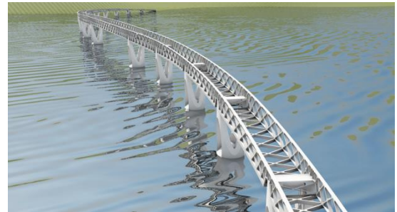
FIGURE 9-5 LATTICE BRIDGE GIRDERS WITHOUT THE TOP
