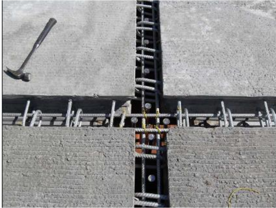
Fig.Ap3.32. Intersection of center line joint and transverse joint prior to filling the joint
