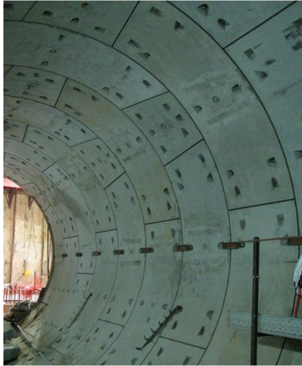
Fig.D19. Close view of segment lining [72]
