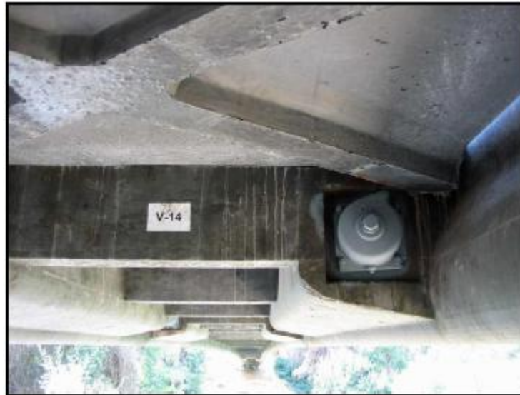
Fig.Ap3.6. Detail of a cross on the underside of deck
