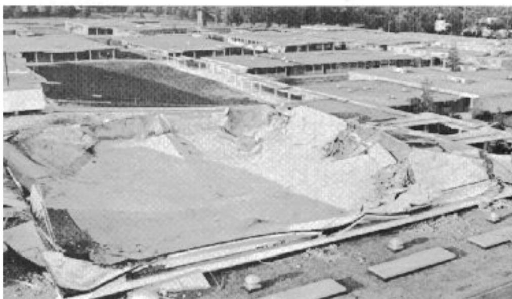
Figure 180. Newspaper photograph of the collapsed hypar shell [81]
