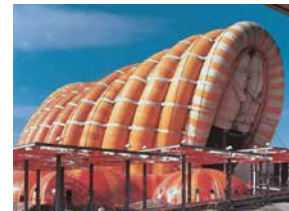
(c) Pneumatic structural system [20].
