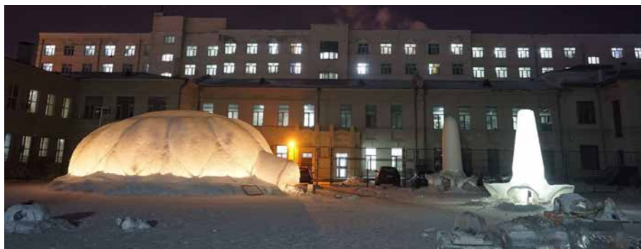
FIGURE 0.5 Three ice composite shells built at HIT, 2016
