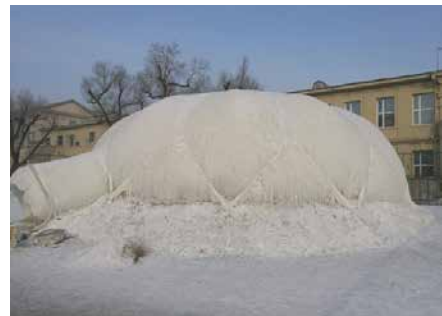
(b) Ice dome after construction.
