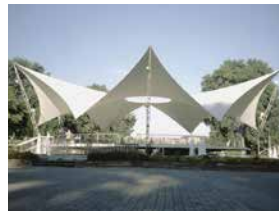
(b) Tension structural system [19].
